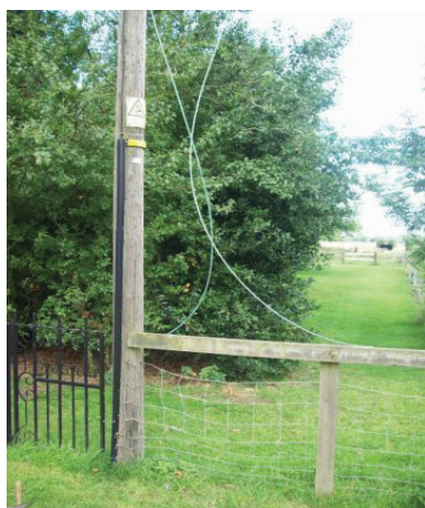
Overhead cable left hanging close to the floor after unwanted interference
